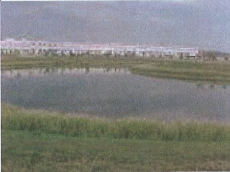
A Detention Pond
