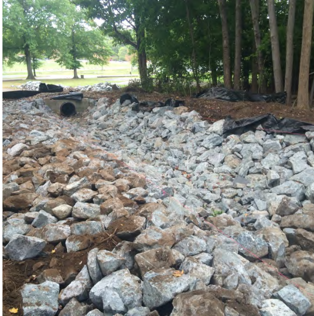
MK-NC-20 Channel Stabilization Construction
