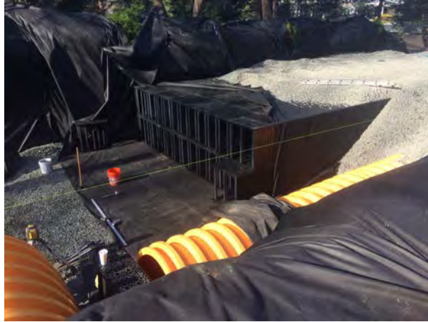
Subsurface Infiltration at B-MU-41
