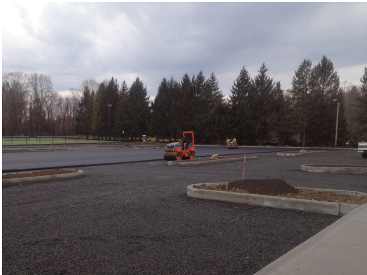
Porous Asphalt Installation: S-MU-09A
