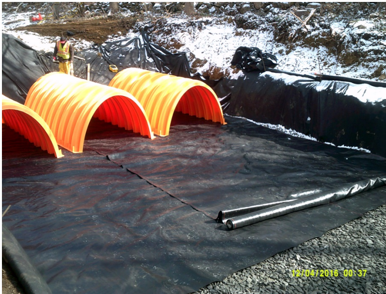
Subsurface Infiltration Construction: B-MU-35
