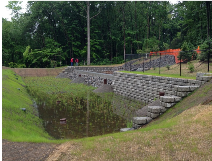
Subsurface Gravel Wetland: SE-POT-01
