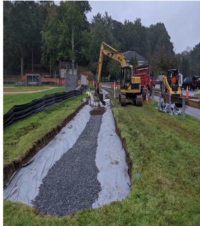
Sand Filter Installation: MK-NC-22
