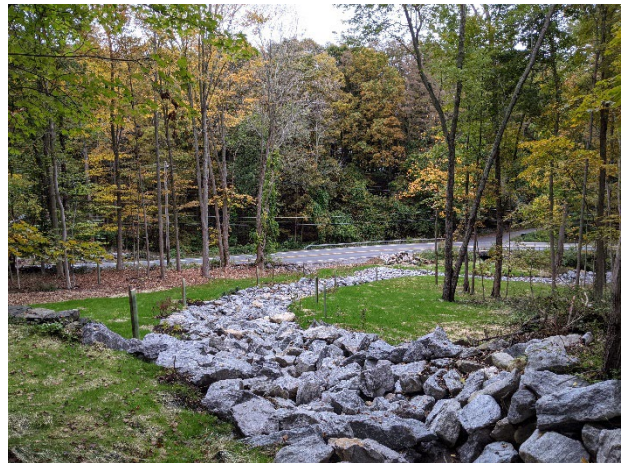
Channel Stabilization: Carmel-CF-601
