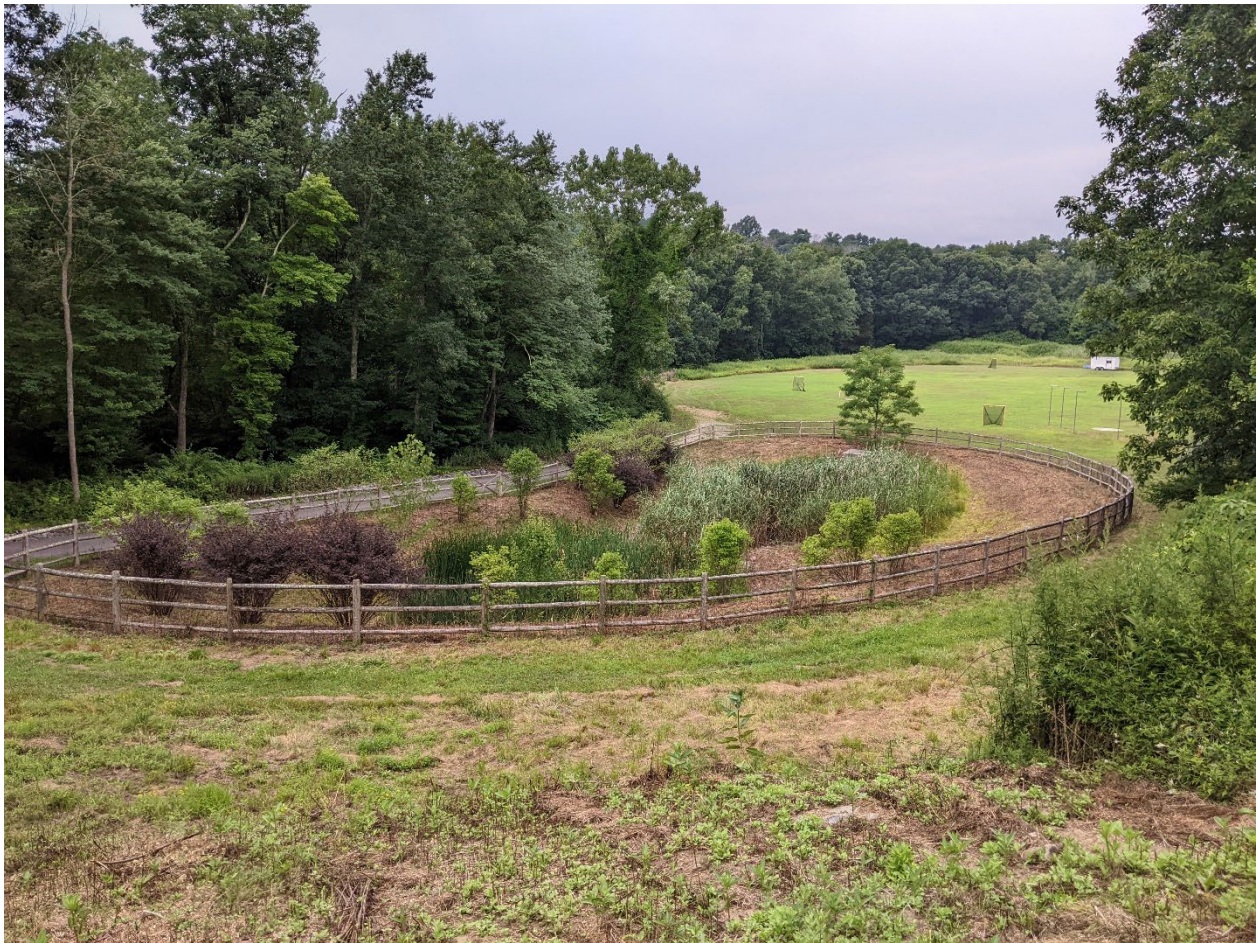
Stormwater Pond – John Jay Cross River, Lewisboro, NY
