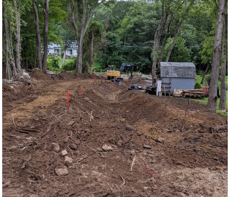
Stabilization Installation: PR-CR-701
