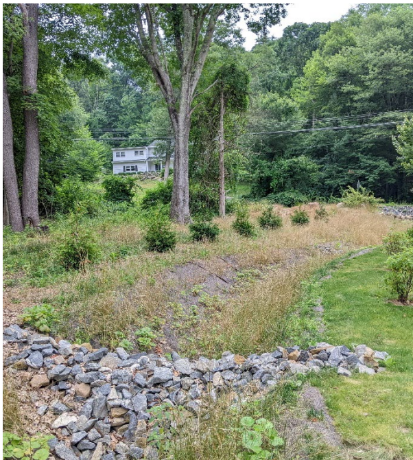
Post Construction PR-CR-701
