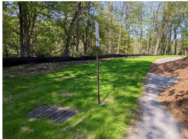
Parking Lot Subsurface Infiltration: L-CR-804
