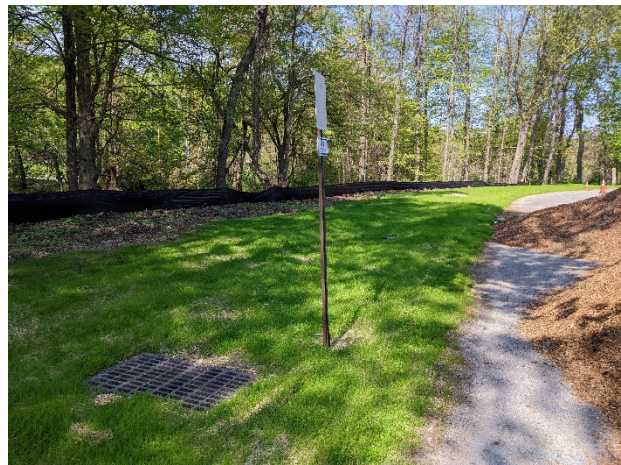
Parking Lot Subsurface Infiltration: L-CR-804
